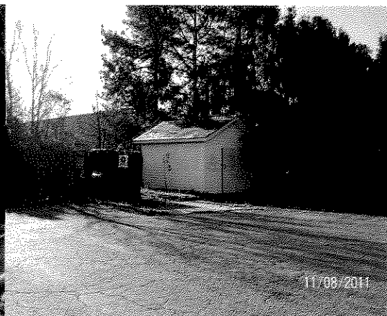
Graffiti Violation After Abatement
