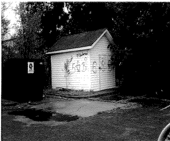
Graffiti Violation Before
