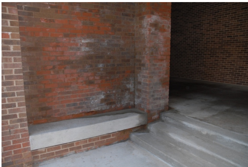
Main Campus Water Penetration Causing Structural Damage & Stains
