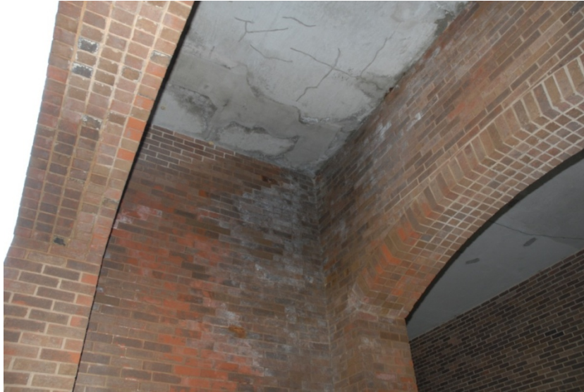
Main Campus Water Penetration Causing Structural Damage & Stains
