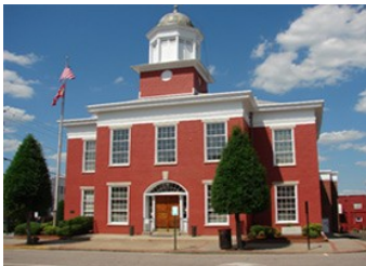
Granville County Court House
