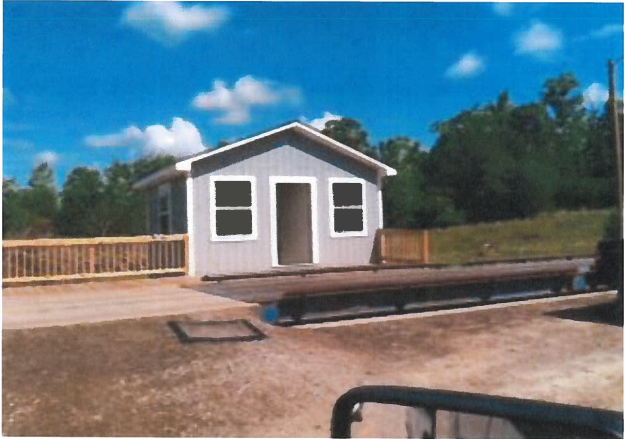
Newly Constructed Scalehouse
