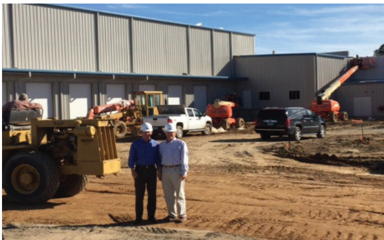
Mike and Lawson Williams at the new M.R. Williams warehouse facility.
